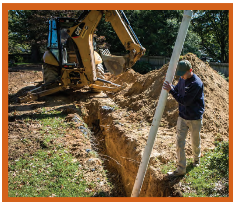
Operator Dan Farrow uses a Cat backhoe to dig a trench for a new septic system.
